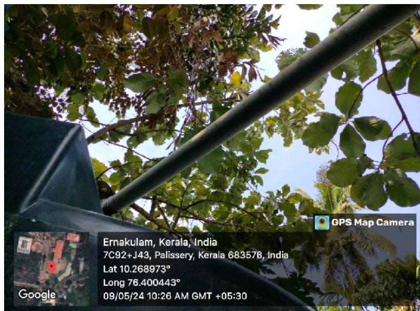
Figure no.3 Connected to water tank
