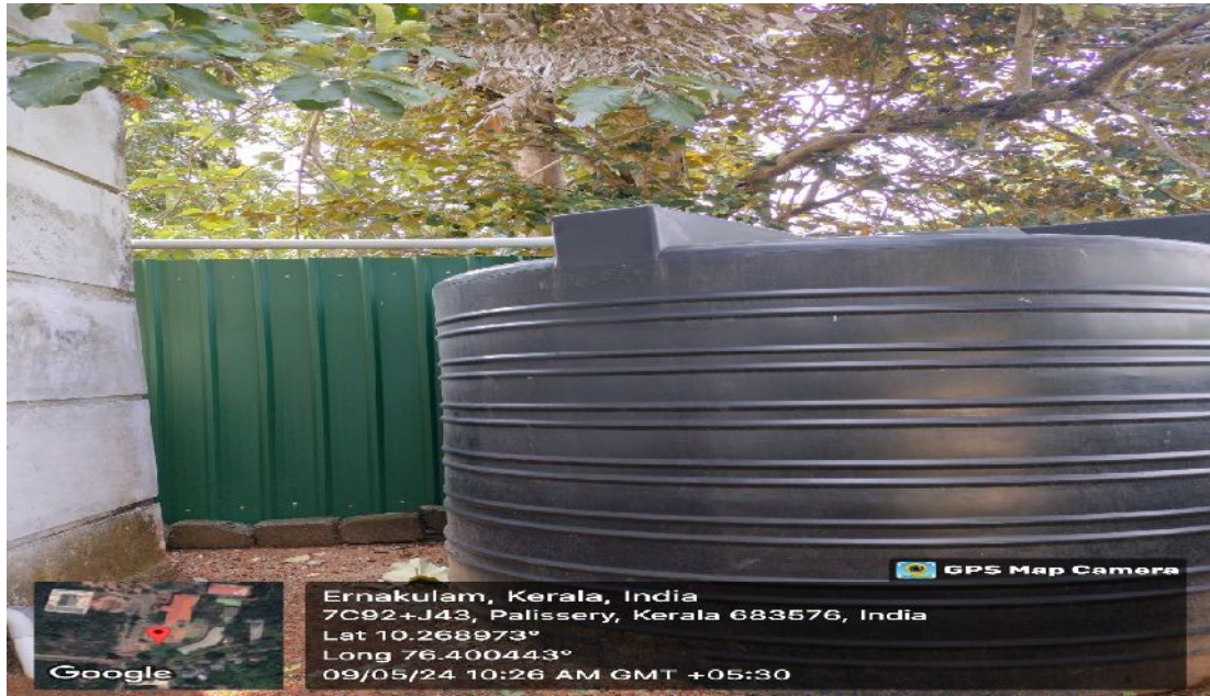
Figure No.4 – Rain water stored in water tanks
