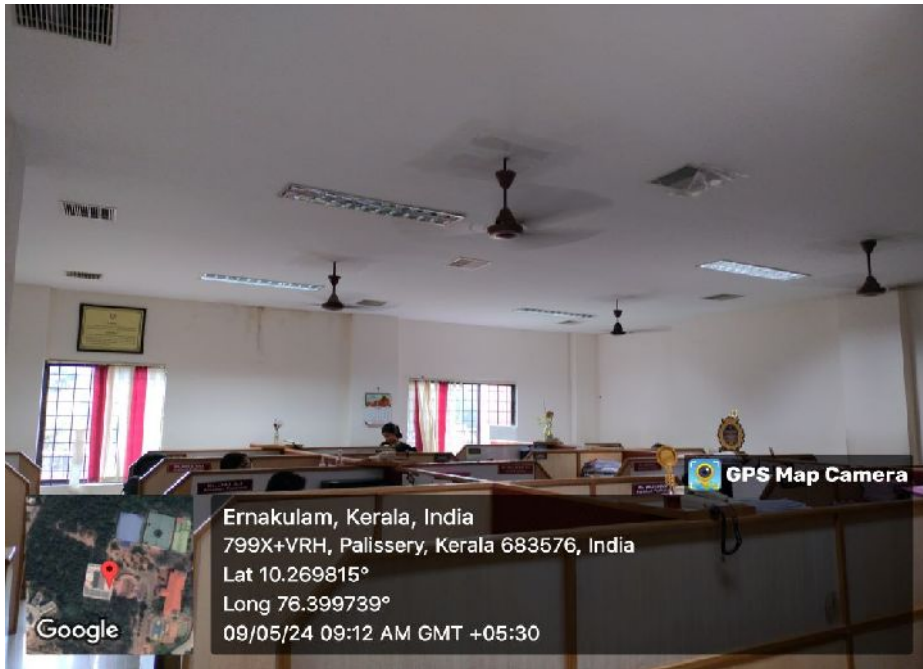
Figure no.10 - Installing Ceiling Fans in Faculty Rooms
